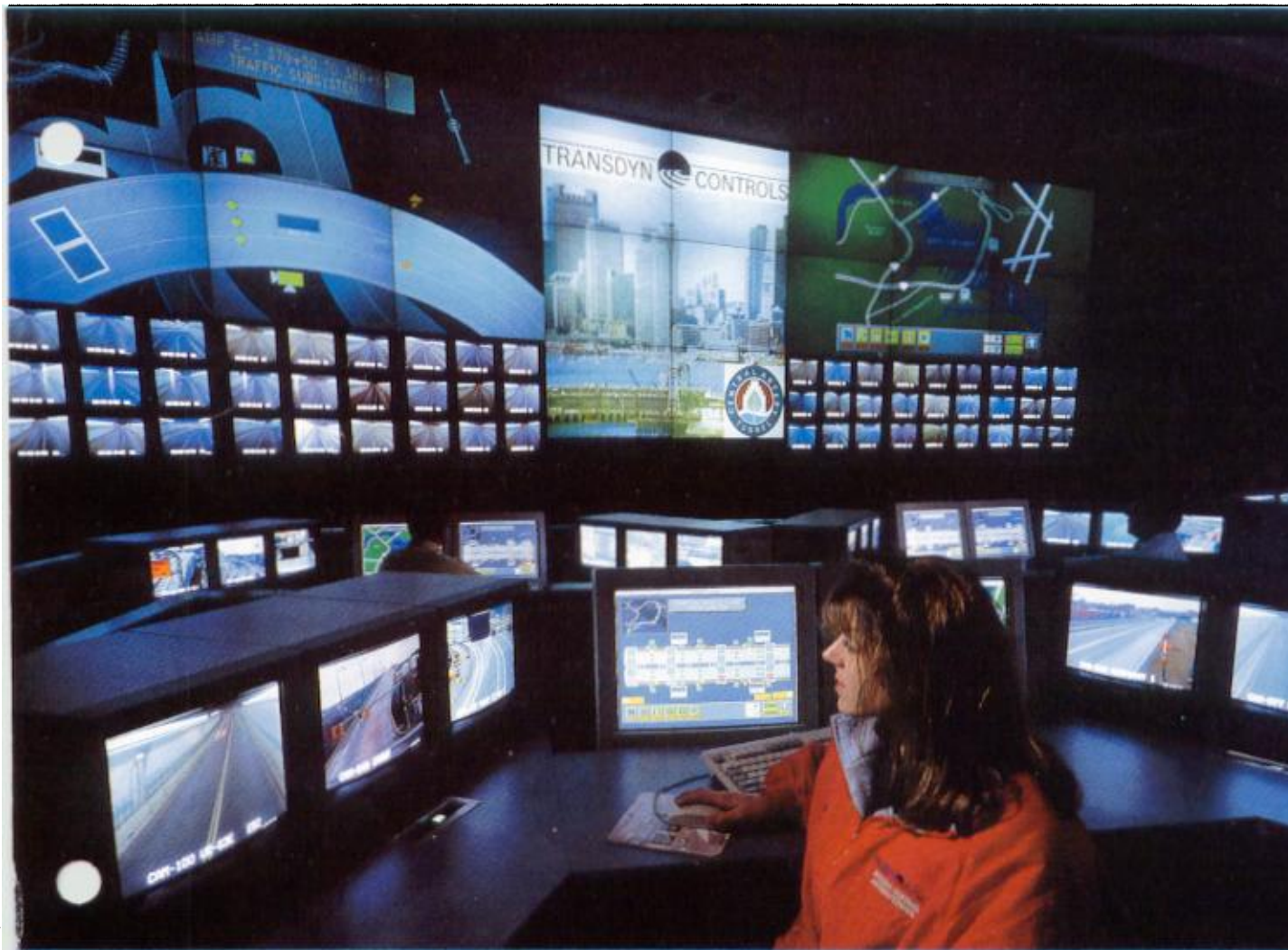
COMPOUND EYE: Operators in the “Star Wars” control center (above) can see every inch of the CA/T system. Along the highway 500 cameras feed images to a wall of monitors; when the computer detects a problem, it switches the video image to an operator’s desktop monitor. The operator can alert drivers to lane closings and speed limit changes using variable message signs (below).
