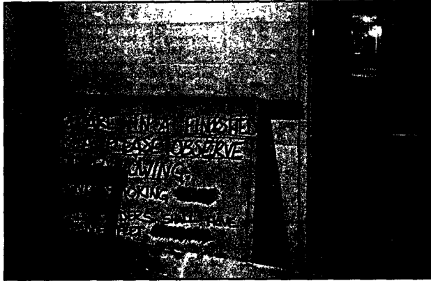
The building is in a strange state of incompletion. In some offices, there are final coats of paint and shelving. In other rooms, the concrete floors have yet to be poured.
