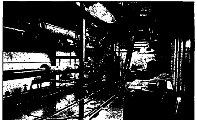
The basement of Building 68 has a massive dual intake ventilation system, redundant pipes, electrical systems, and water lines. The upstairs laboratories are already well apportioned with cold rooms and autoclaves. This place is a biologist's dream come true.
