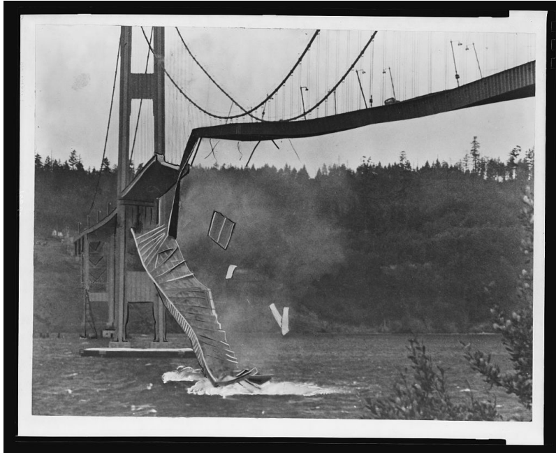
Tacoma Narrows Bridge Collapse (1940)
